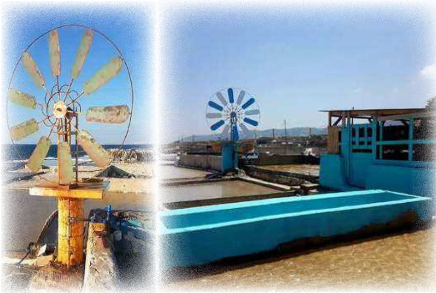
Figure 165. The windmill, a characteristic feature of these saltworks and a tourist attraction, before its restoration (left) and once restored for water pumping, next to the spa pool (right). ©Georges Sleiman/Evaura
