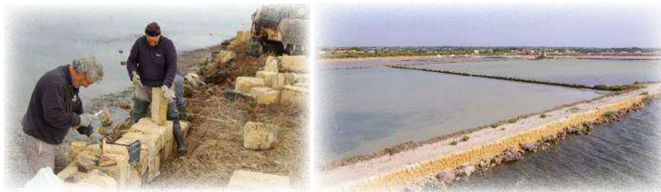
Figure 19. One of the embankments recovered in the Ettore and Infersa salina (Italy) within the MedArtSal project pilot actions (above) and the rebuilt and reinforced wall in the San Vicente salina (Spain; below). ©MedArtSal project
