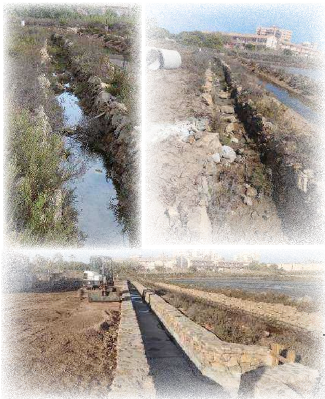
Figure 145. The salt pan's canal before the intervention (top left); during the renovation (top right) and after the renovation work (below). ©ANSE
