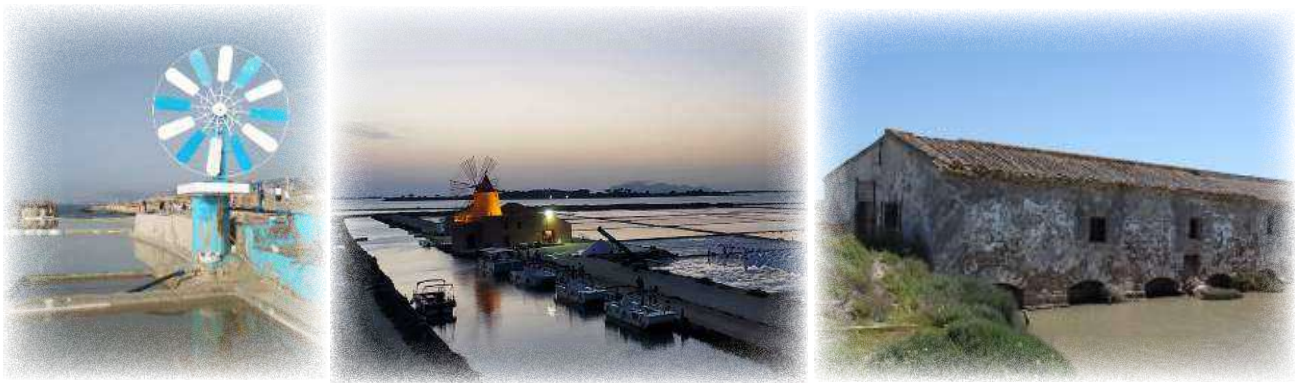
Figure 75. Windmill in Georges Salinas, whose function was to bring water from the sea into the ponds (Lebanon; left). Landscape in Salina Ettore e Inversa (Italy; middle) with a salt windmill. Abandoned tide mill in the Bahía de Cádiz Natural Park (Spain). ©H.Clavero (left and right) and T.Campisi (middle)
