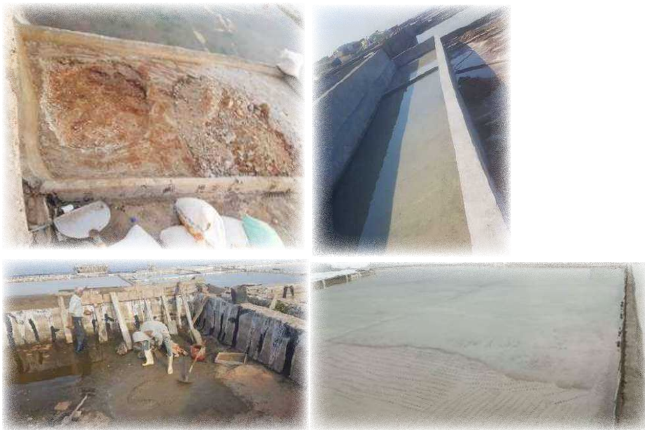
Figure 163. Salina pond rehabilitation (top, and bottom left). After work (bottom right). ©Georges Sleiman/Evaura
