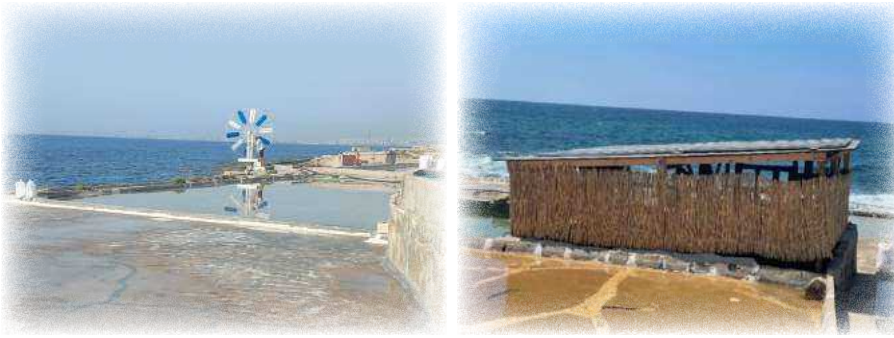
Figure 21. Traditional windmill repaired in Sleiman Sleiman Salinas (left). Solar panels installed in George Sleiman Salinas (right) (Lebanon, MedArtSal pilot actions). ©T.Campisi (left) and MedArtSal project (right)
