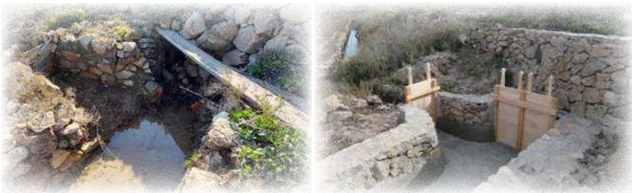
Figure 146. The sluice gates before and after the reconstruction. ©ANSE
