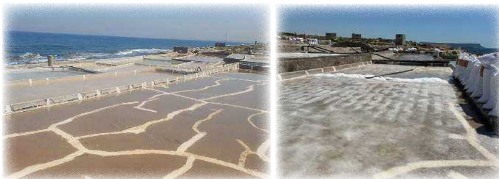
Figure 160. Salt ponds rehabilitation (left). Salt production in rehabilitated salt ponds (right), Blanc Sel Salinas, Anfeh, Lebanon. ©Jessica Najjar/Blanc Sel Salinas
